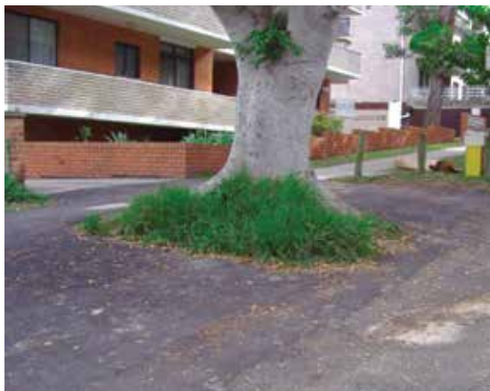
Concrete kerb, gutter and footpath replaced with bitumen to minimise damage to tree roots
