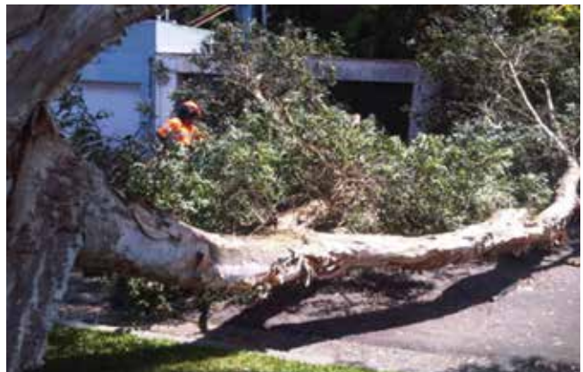
Emergency work to a street tree
